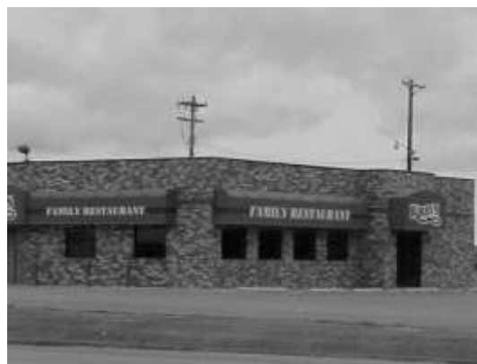
Sign, Architectural Canopy Sign, Awning or Canopy
